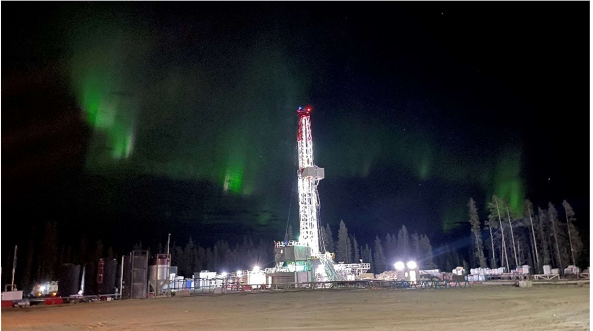
Ensign Rig #401 has been drilling for Peyto for over 12 years.
